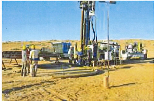
For a recent project in South Africa's Northern Cape, a new Mincon reverse-circulation (RC) system was used, successfully drilling to 1,019 m in just nine days
