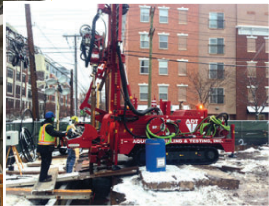
Fraste for extracting high-quality soil samples
